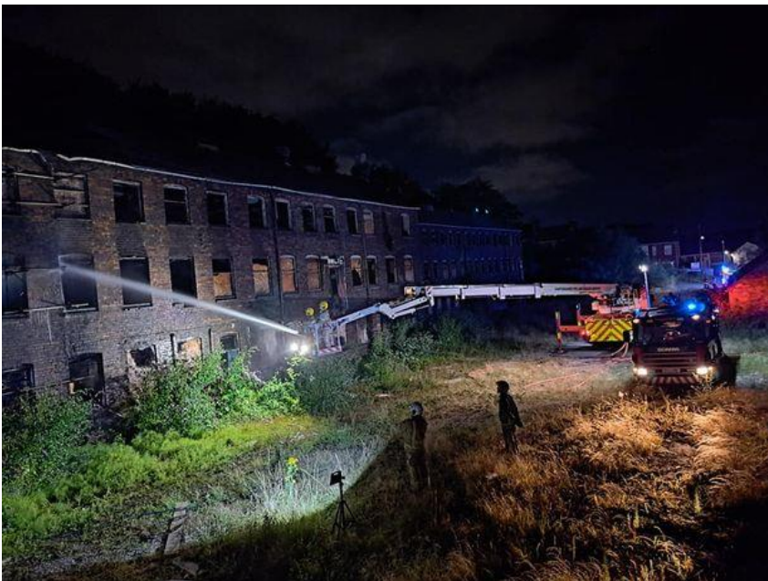
Firefighters tackling the blaze at the former Falcon Works in Stoke (Image: Staffordshire Fire and Rescue Service)
